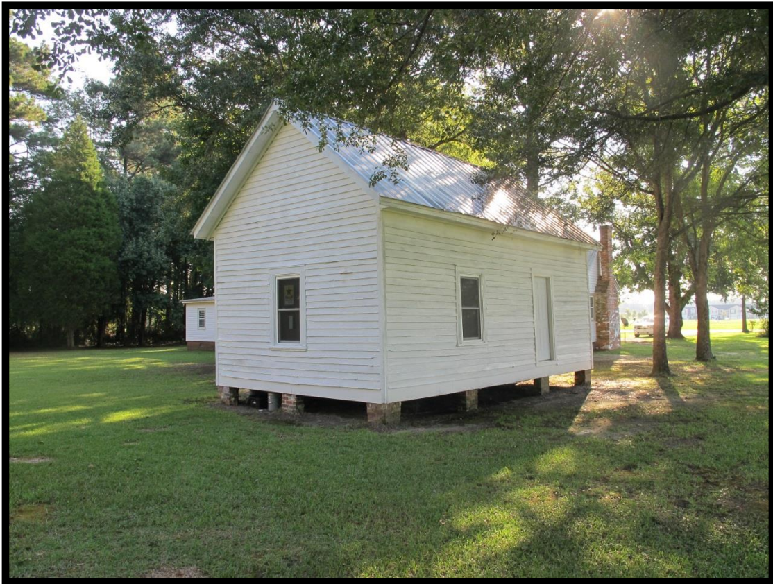
Figure 14: Noah Forbes, Sr. House (# 1), Forbes Schoolhouse Looking Northeast.
