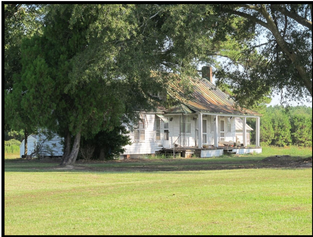
Figure 21: View of the Caleb Smith House (PT0186), Looking North.
