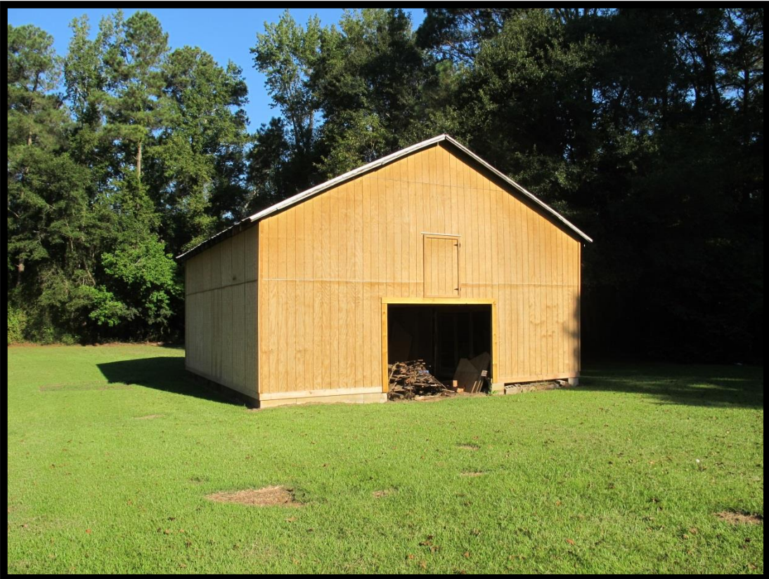
Figure 10: Noah Forbes, Sr. House (# 1), Barn Looking Northwest.
