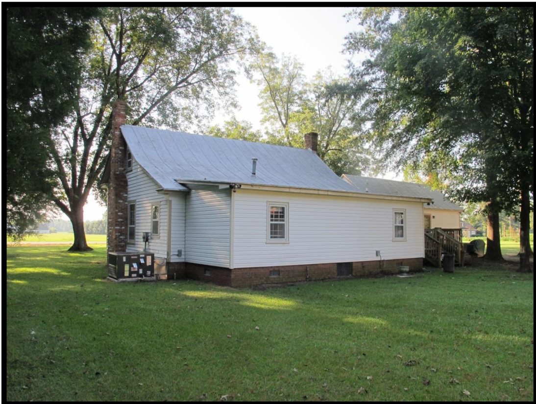
Figure 6: Noah Forbes, Sr. House (# 1), Looking South.
