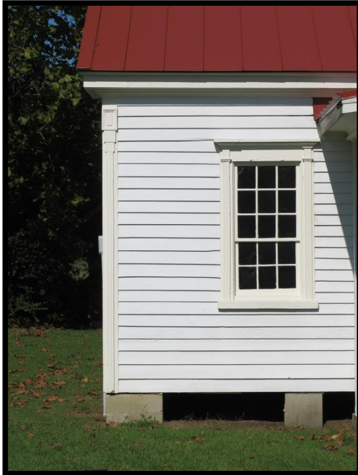
Figure 24: Detail of the Thomas Adrian Savage House (PT0316a), Showing the Window Surround and the Corner Board.
