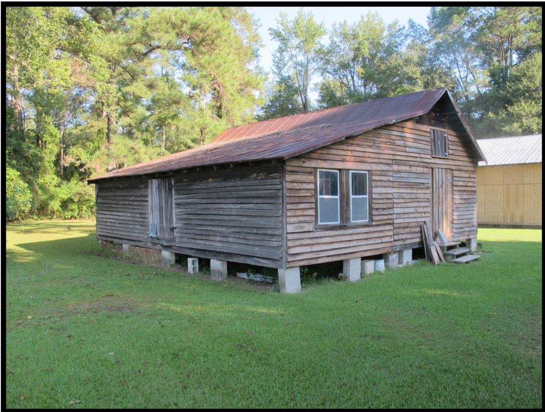
Figure 12: Noah Forbes, Sr. House (# 1), Outbuilding Looking Northwest.
