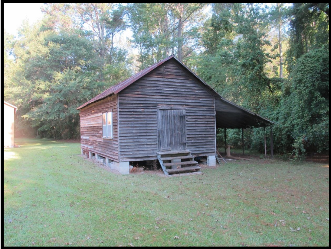
Figure 9: Noah Forbes, Sr. House (# 1), Outbuilding Looking Northwest.
